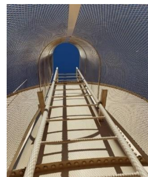
Ladder to top of a tank
